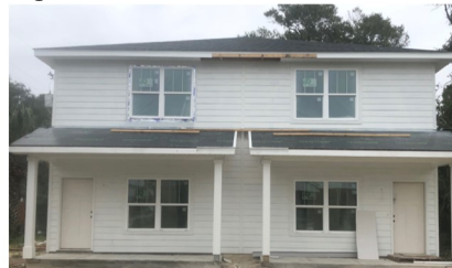
Townhomes in progress on this Lot 48 & 58 North M Street
