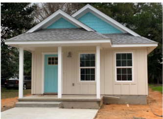
Home in progress on this Lot 2210-A North Tarragona Street
